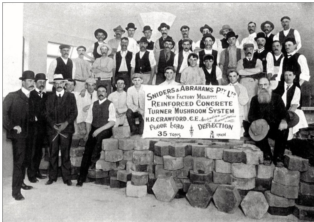
SNIDERS & ABRAHAMS PROP. LTD.—FACTORY, MELBOURNE. Test Load on Second Floor:—Loaded 16 ft. square (weight of workmen not included). Columns, 18 ft. 6 in., centre to centre.
