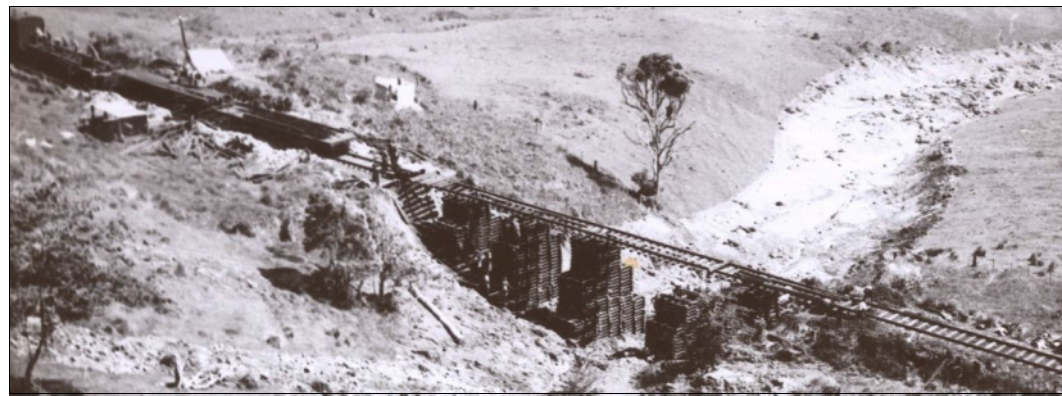
A train delivers the bridge beams to the northern end of the work.
