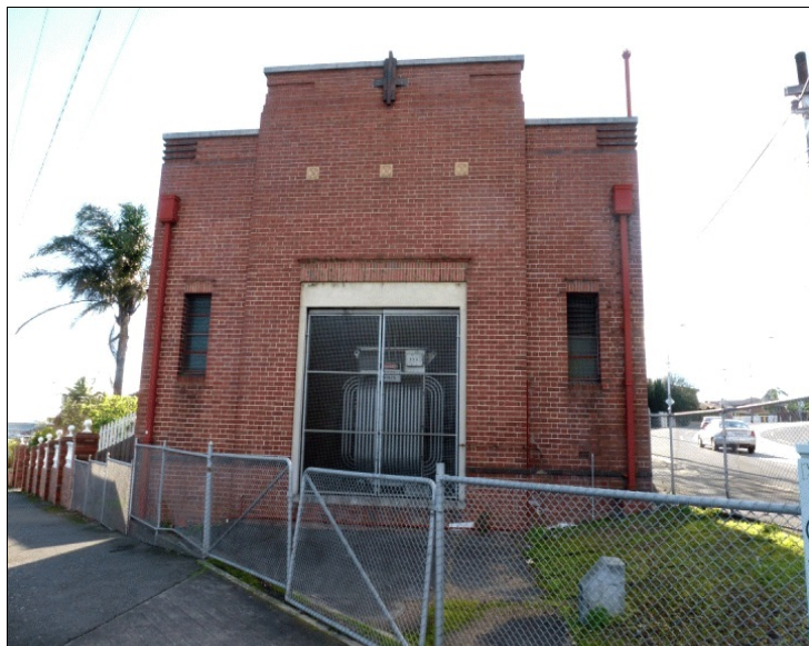
The Brunswick West Tramway Substation, viewed from the corner of Dawson Street (left) and Melville Road (right). Photo: Miles Pierce, 2014.
