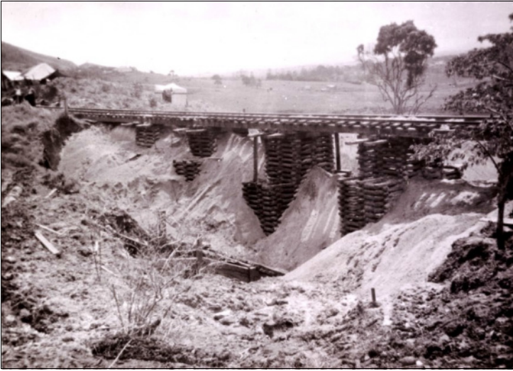
Once the railway was re-opened the task of rebuilding the embankment was straightforward using bottom dump wagons to tip sand through the track and the sleeper towers. SARA NRS17420_2_1684_140P
