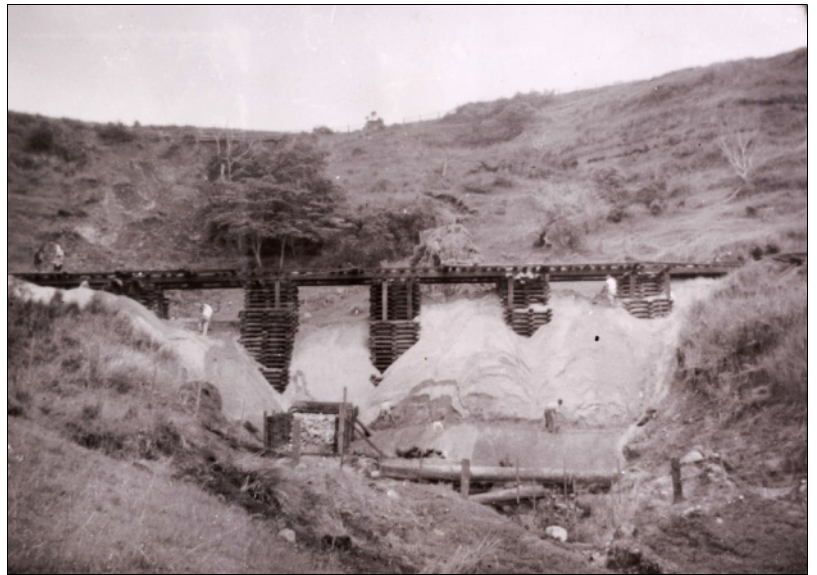
Provision for water flow through the new embankment is provided by a rock filled timber box drain (see at left of the gully base). It was expected to ultimately rot and collapse. SARA NRS17420_2_1684_140Q
