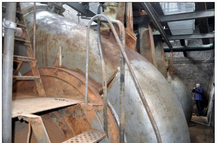
Main pump casing (foreground), the engine behind it, and the 2 nd pump casing just visible behind that – all before repainting. In the background is Paul Stephens, President of ISSSES, on a visit to Australia. Image: Owen Peake.
