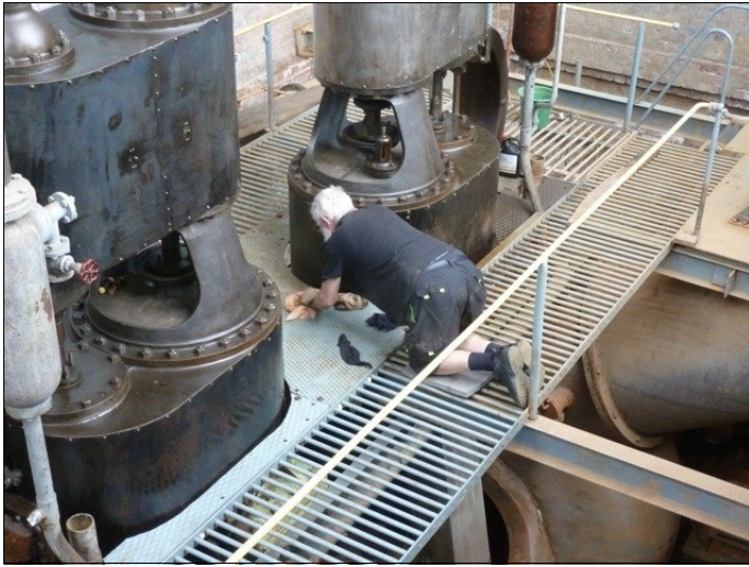
The author cleans floor plating on the operating floor prior to painting while kneeling between the two sets of high & low pressure cylinders. Part of a pump can be seen below the floor grid. Image: Miles Pierce, Sept 2013.
