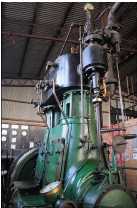
Thompson 100 kW triple expansion steam generating set. Image: Owen Peake
