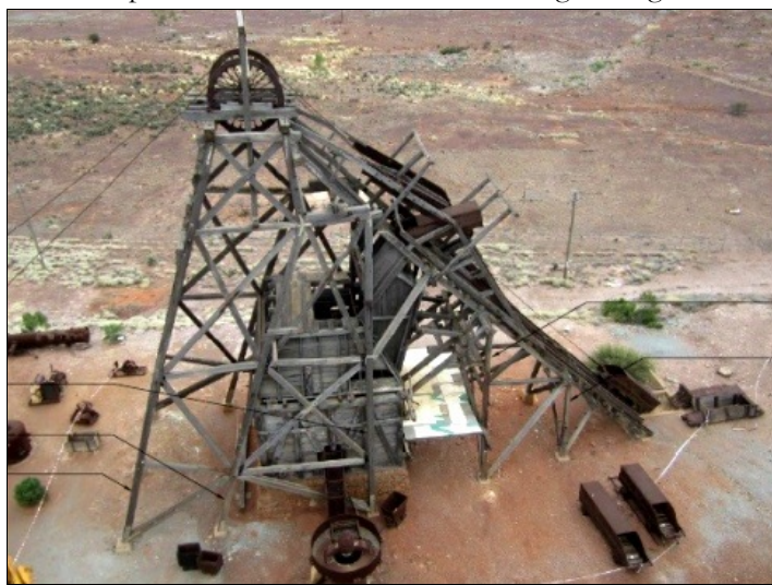
The Sons of Gwalia headframe in 2012. Image: Martin Silk, Intelera Consultants.
