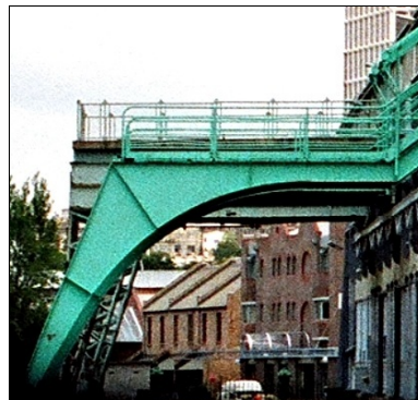
East elevation of Wharf Shed 6, looking south from the transept. Shows a gantry rail on the wall and a welded gantry platform in the distance. Two lattice girder platforms are just visible behind it (see detail). Image: M.Doring, Dec.1987.
