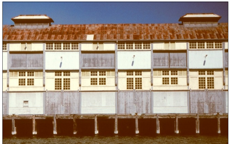
Wharf shed 9 viewed from the west. Shows typical wall panelling with sliding doors. Image: M.Doring, November 1990.
