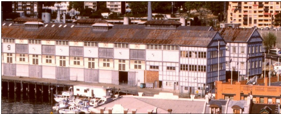
South end of the Finger Wharf seen from the Domain. Note the set back gable roof of the central roadway just visible between the south ends of sheds 9 (near) & 6 (far). Image: M.Doring, 1988.
