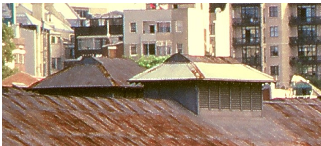
Roof vents over Wharf Shed 9 & centre roadway. Image M.Doring, 1988
