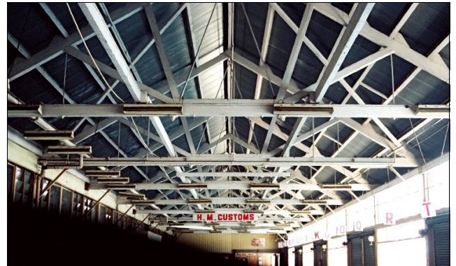
Roof structure over Wharf 7 shed, looking north.
