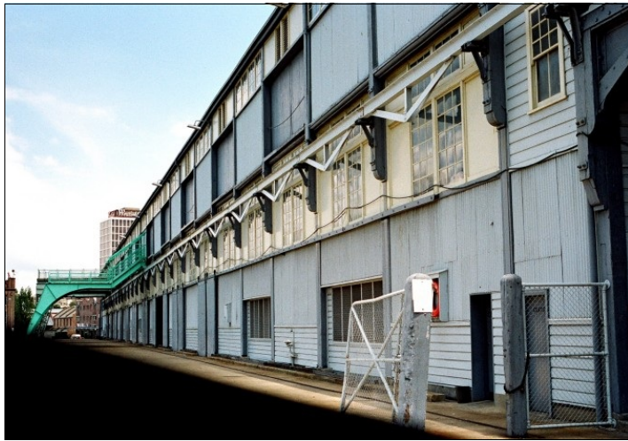
East elevation of Wharf Shed 6, looking south from the transept. Shows a gantry rail on the wall and a welded gantry platform in the distance. Two lattice girder platforms are just visible behind it (see detail). Image: M.Doring, Dec.1987.
