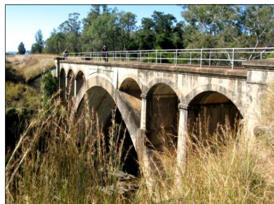
Chowey Bridge over Deep Creek. Image: Brian McGrath
