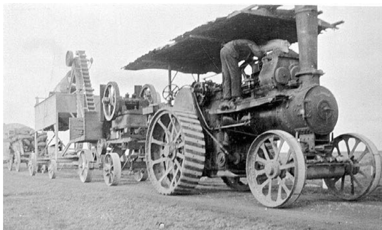
Traction Engine, Grenville, Victoria. Traction engine towing belt driven farm machinery.
